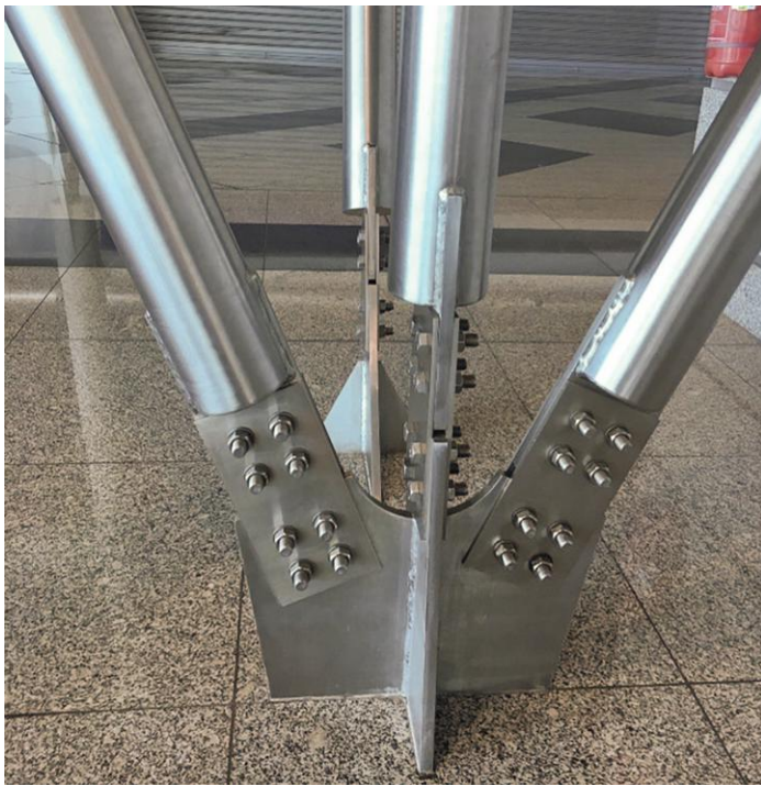
Bracing connection in a stainless steel canopy at Porto Airport, Portugal. Photo on right courtesy of TriPyramid Structures, Inc.
