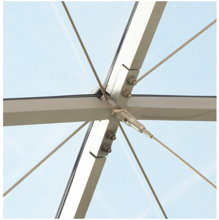
Bracing connection in a stainless steel canopy at Porto Airport, Portugal. Photo on right courtesy of TriPyramid Structures, Inc.
